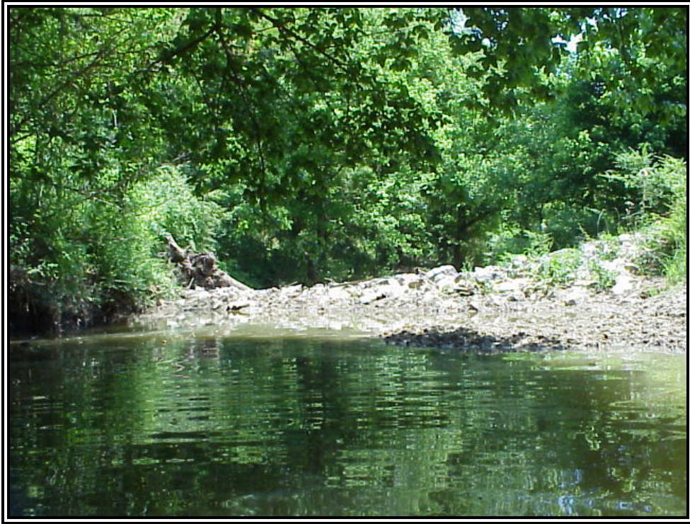
Figure 3.2 Channel Obstruction within Town Creek segment 2
